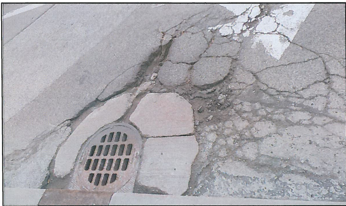
Photo 7 – Deficient asphalt wearing surface and settled catch basin in the westbound lanes of Prospect Avenue in Unit 14
