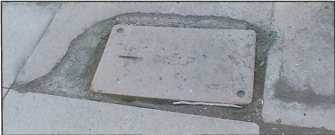
Photo 16 - Typical pull box with missing caulk sealer
