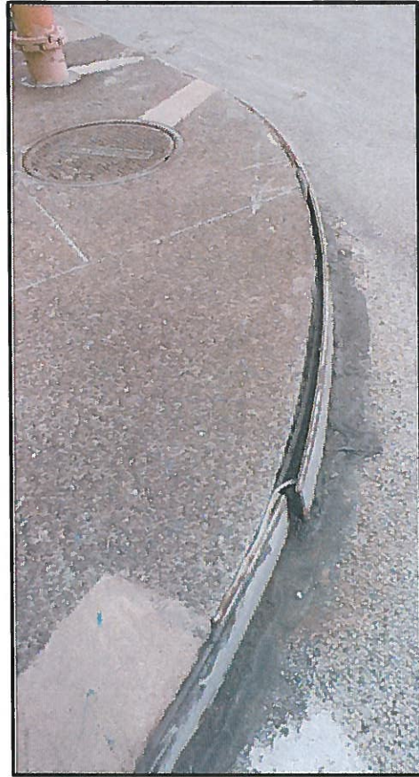
Photos 14 & 15 - Typical loose and missing curb plates
