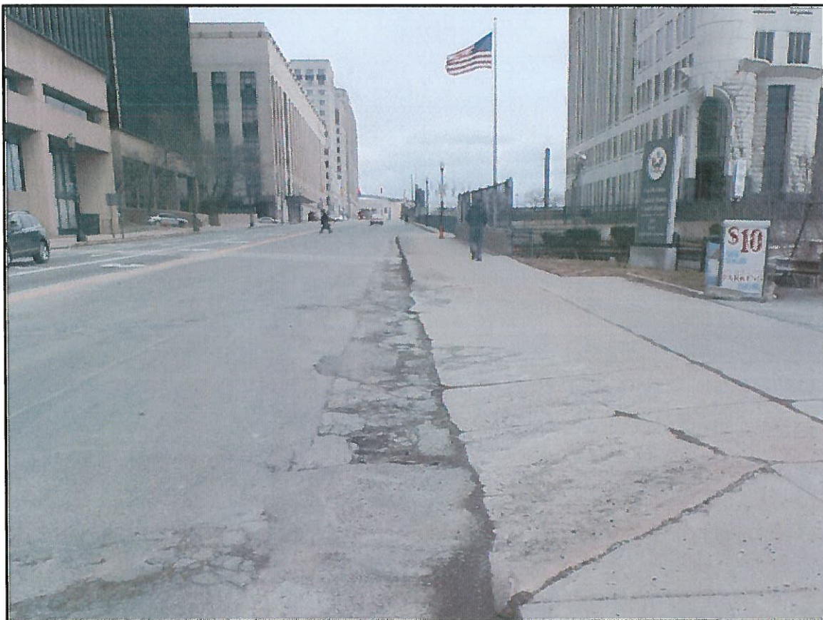
Photo 6 – Deficient asphalt wearing surface in the eastbound lanes of Prospect Avenue in Units 14 & 15
