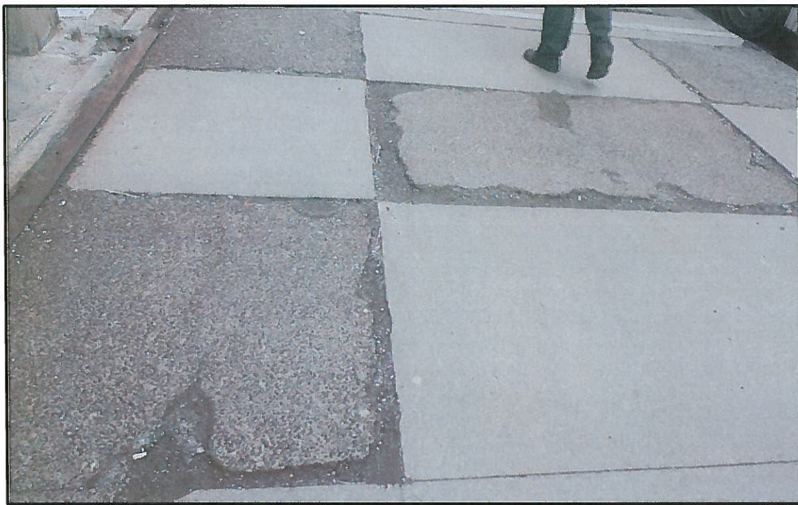
Photo 8 – Typical deficient decorative aggregate sidewalk panels
