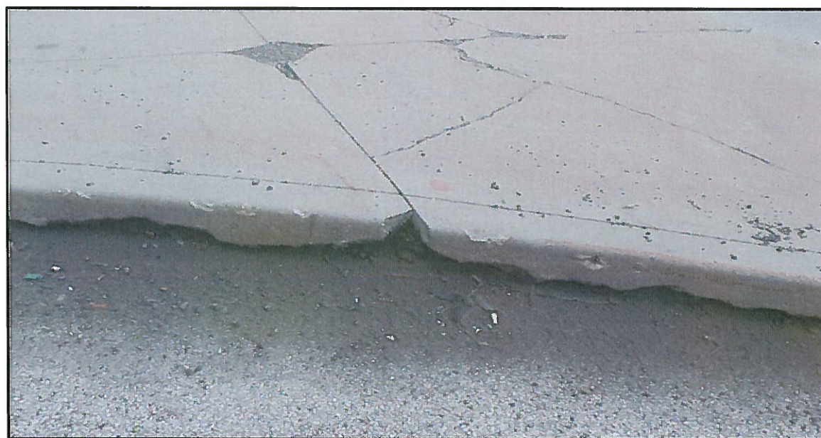
Photos 12 & 13 – Severely undercut curbs at the concrete island at the east end of Huron Ave.
