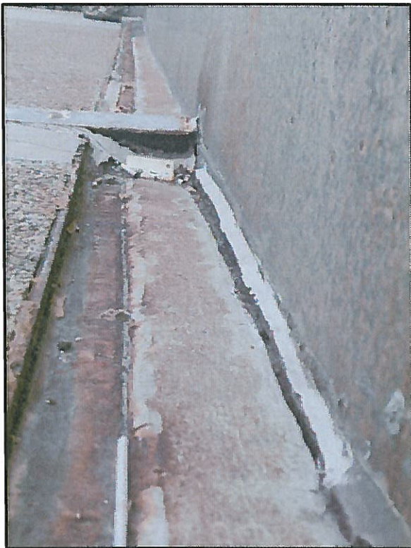
Photo 8 - Typical growth of decorative aggregate sidewalk panels
