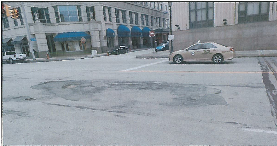
Photo 4 – Deficient asphalt wearing surface in the westbound lanes of Prospect Avenue in Unit 5
