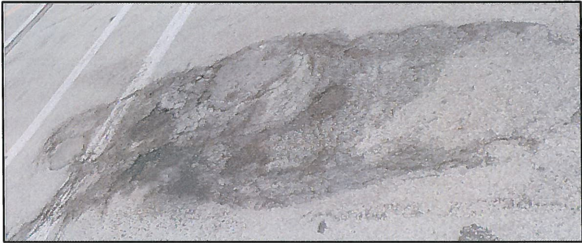
Photo 5 – Deficient asphalt wearing surface in the westbound lanes of Prospect Avenue in Unit 5
