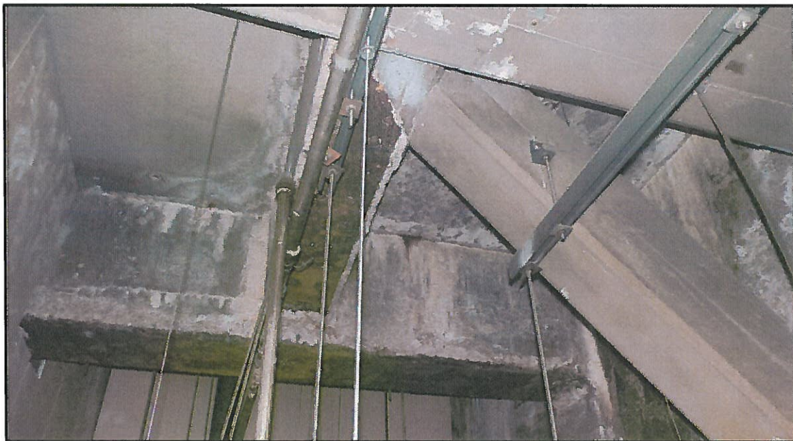
Photo 2 – Active leak in Unit 6, showing typical beam corrosion after removal of fireproofing concrete
