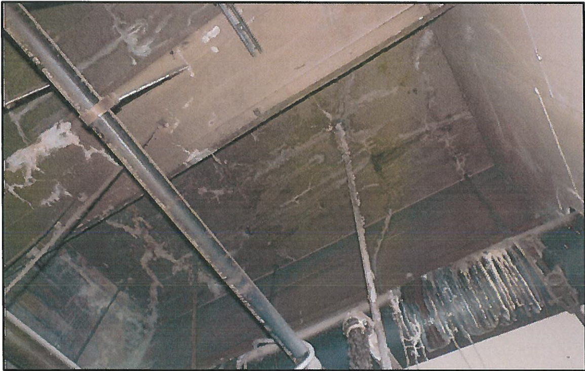
Photo 3 – Active Leak in Unit 26, showing typical map cracking in deficient deck locations
