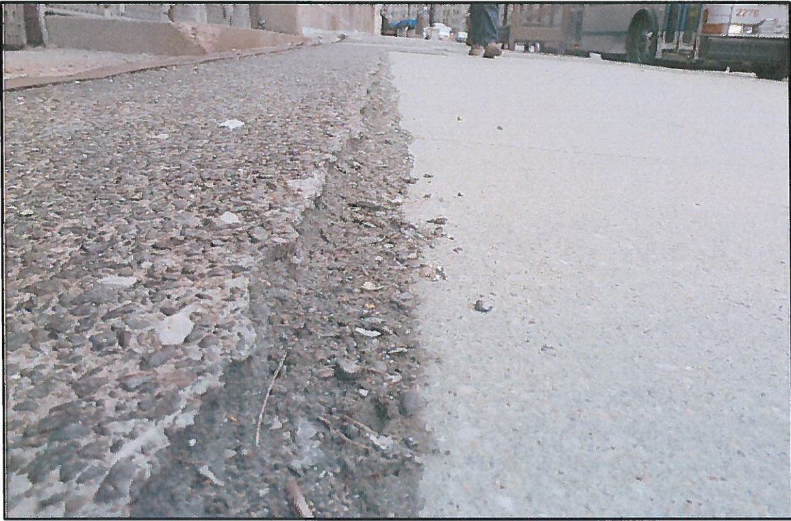
Photo 8 - Typical growth of decorative aggregate sidewalk panels
